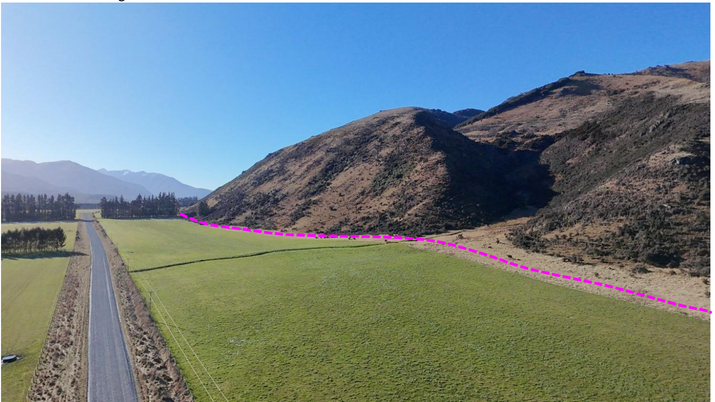
13.8km. Looking north along base of hills
