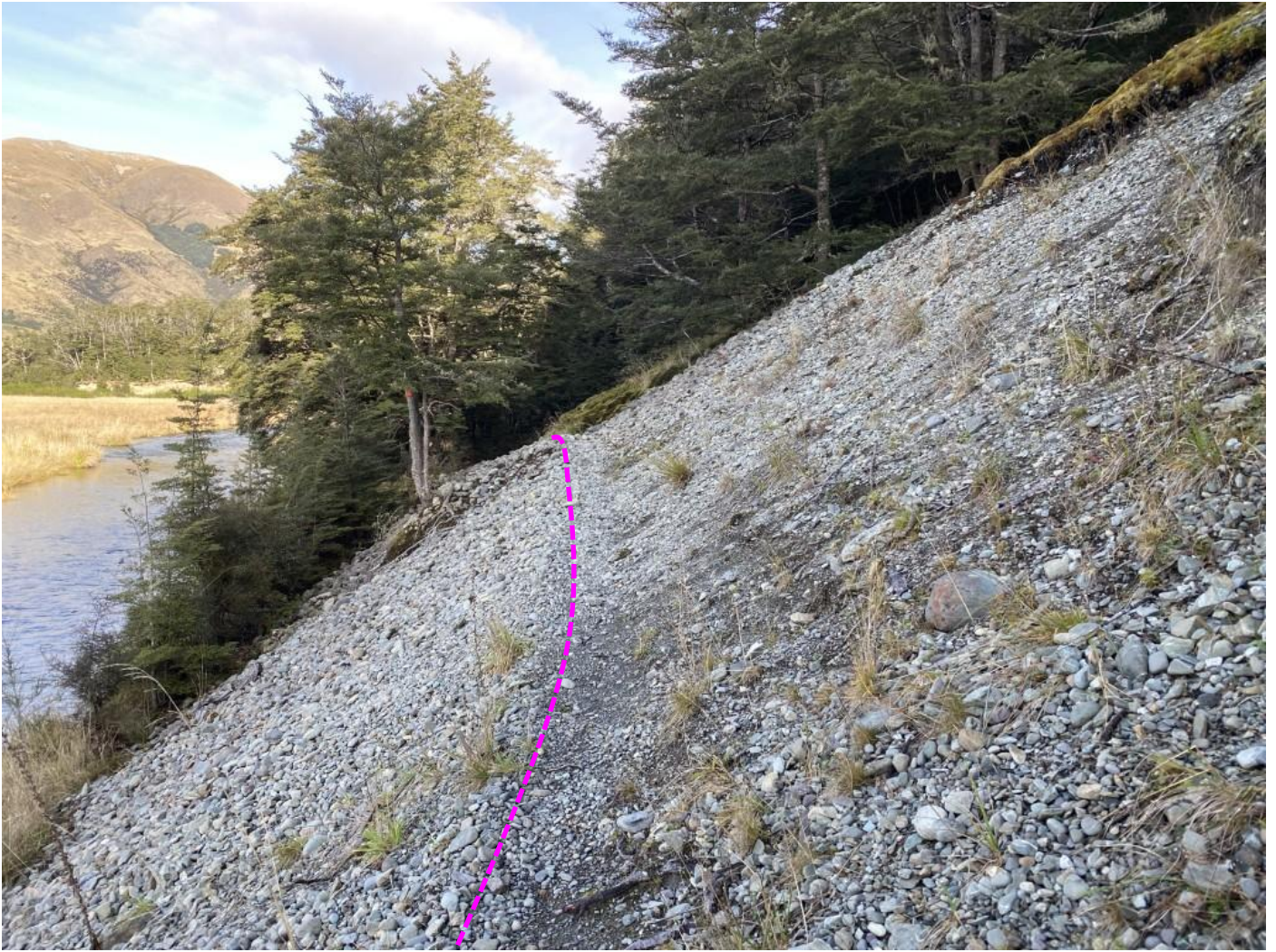
Gravel banks near Kiwi Burn Bridge. Well-designed retaining will manage maintenance risk here.
